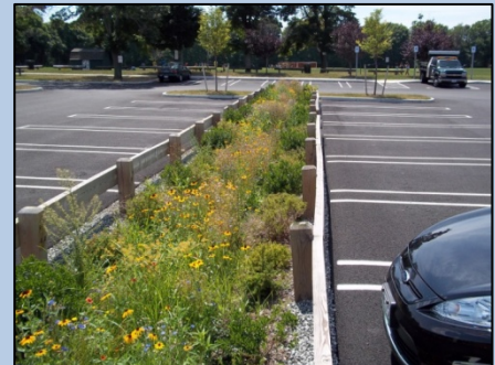
Bio-retention system for stormwater runoff from the parking lot at Bristol Town Beach
