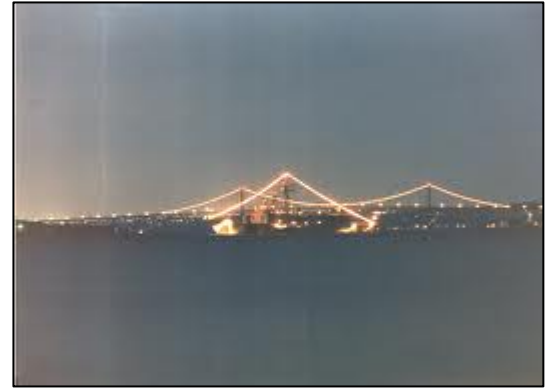
Mt. Hope Bridge
