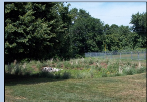
Vegetative infiltration basin at Bristol Town Beach
