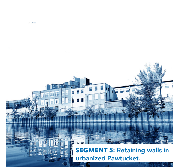
SEGMENT 5: Retaining walls in urbanized Pawtucket.
