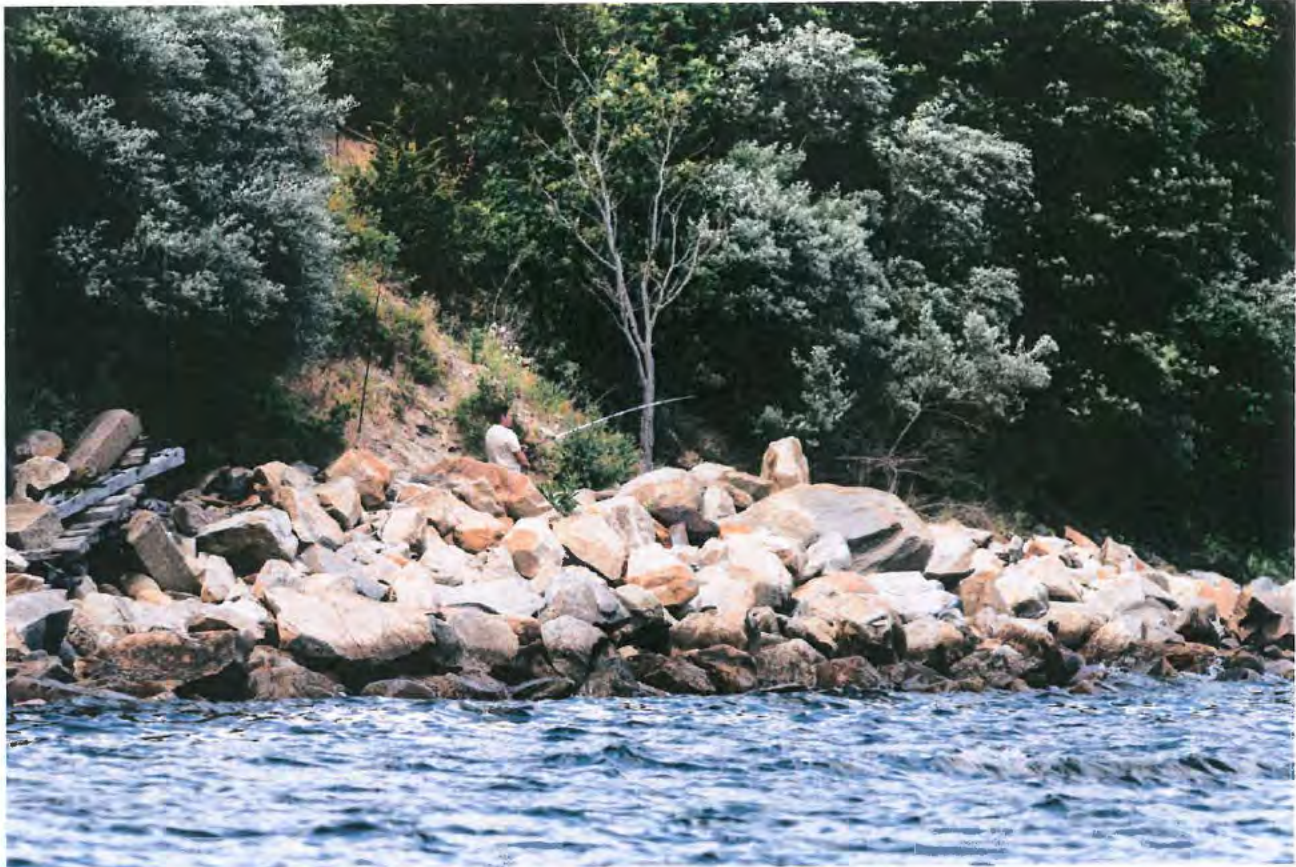
Fisherman using area immediately North of illegal wall. This area is no longer accessible to the public from the South.
