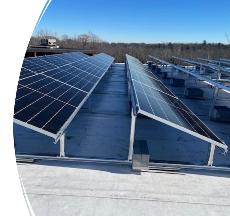
Thermoplastic polyolefin(TPO) roof. High density board (cover board) adds life to the roof. TPO is many times stronger and durable than a rubber roof (EPDM). New white roofs with bifacial modules qualify for a 30% Investment Tax Credit.
