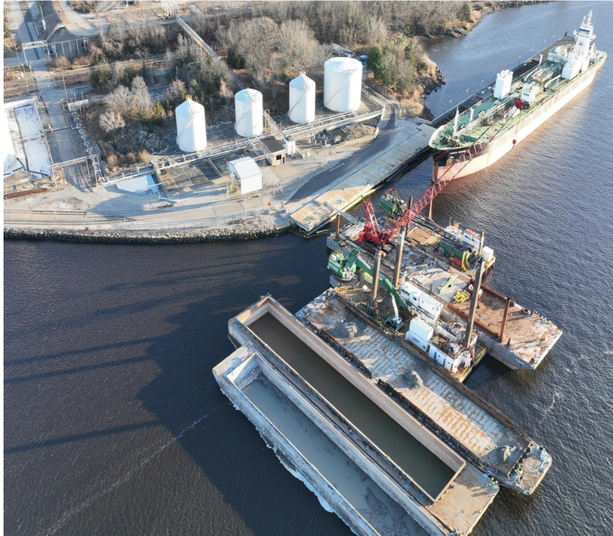
Reconstructed pier with Montville powerplant and Transmission lines
