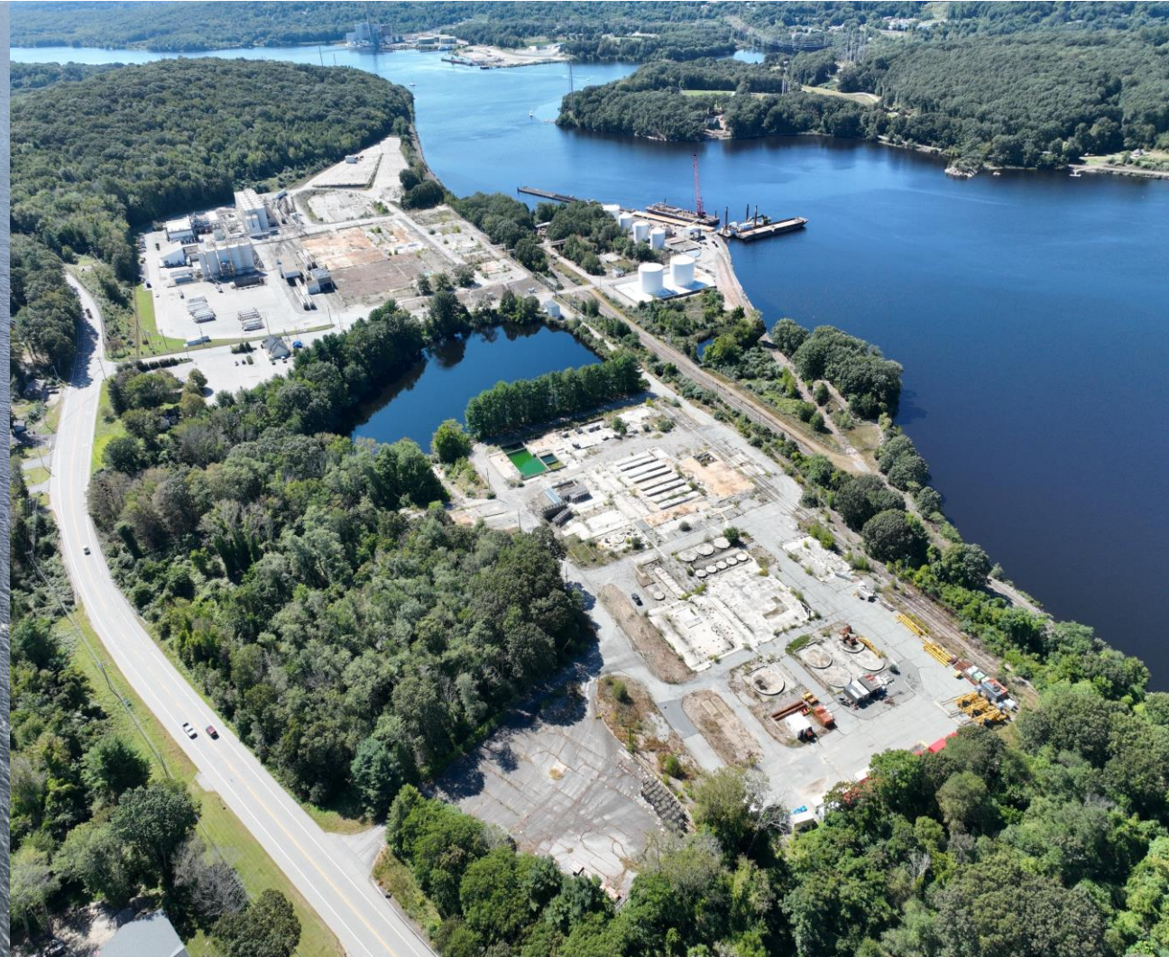
Amsty and the remains of concrete slabs
